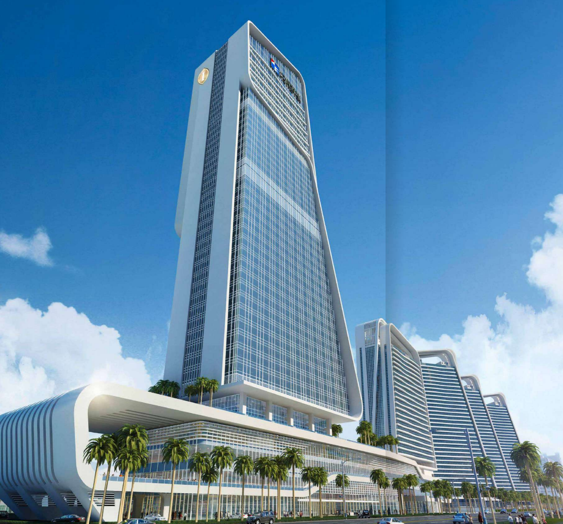
Zhuhai, Yanheng Land Commercial Complex
